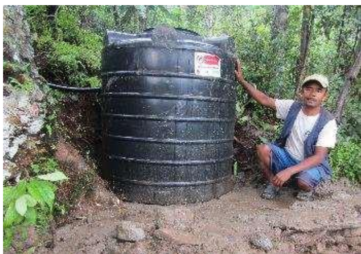
Poly-tanks connected with natural water wells for storage of drinking water during dry seasons
