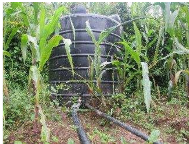
Poly-tanks connected with natural water wells for storage of drinking water during dry seasons
