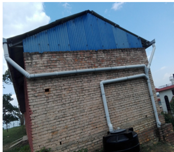
6 the pipelines to collect the rainwater
